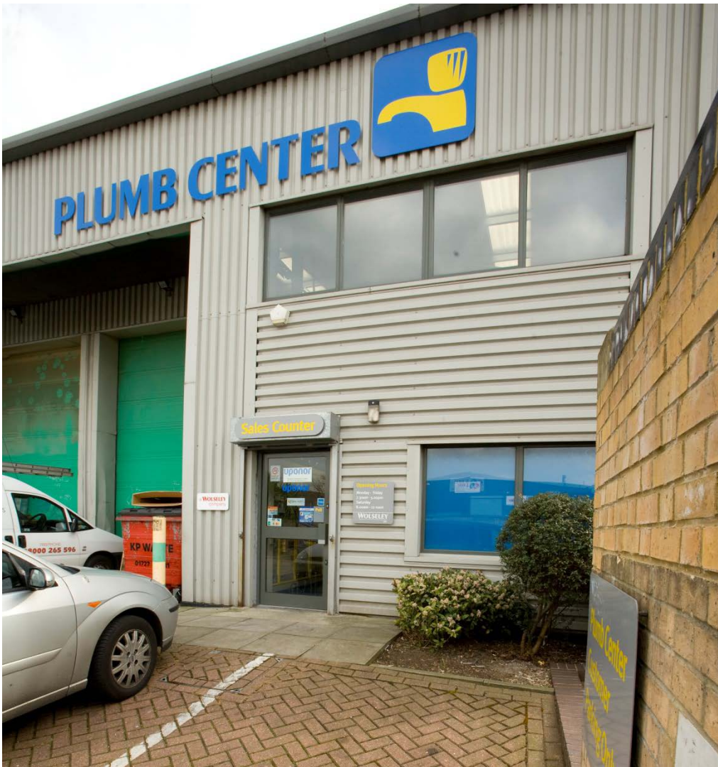
The Apsley Centre, London NW2
